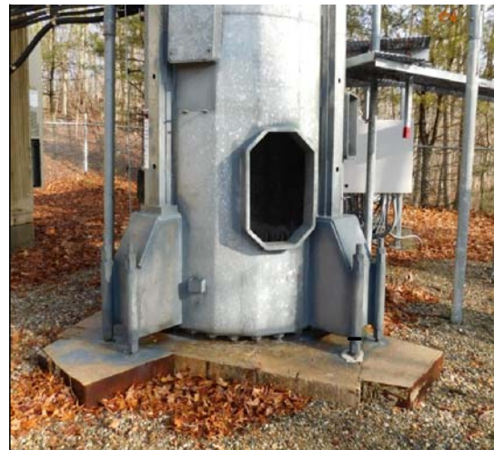
TOWER BASE/FOUNDATION PHOTO
