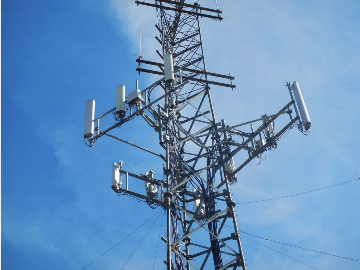
Photo 1: Photo illustrating the Tower with Appurtenances shown.
