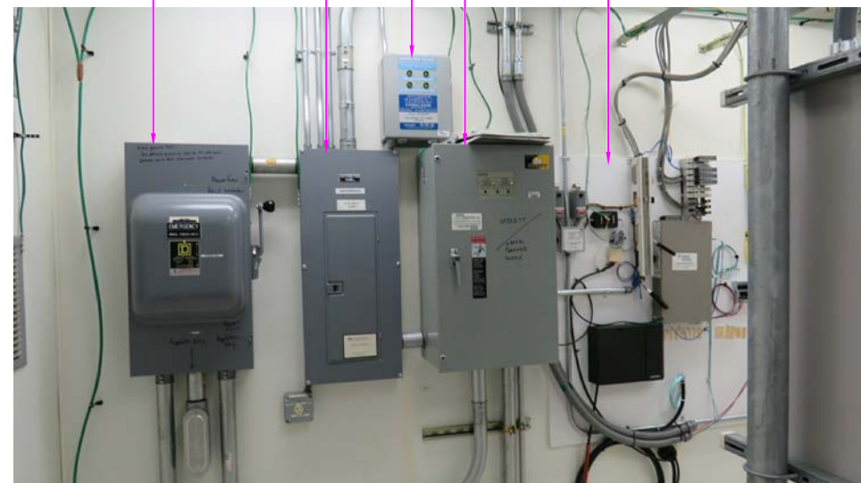
IMAGE SOURCE: PROTERRA 10/14/2017 (VIEW FROM WEST)
