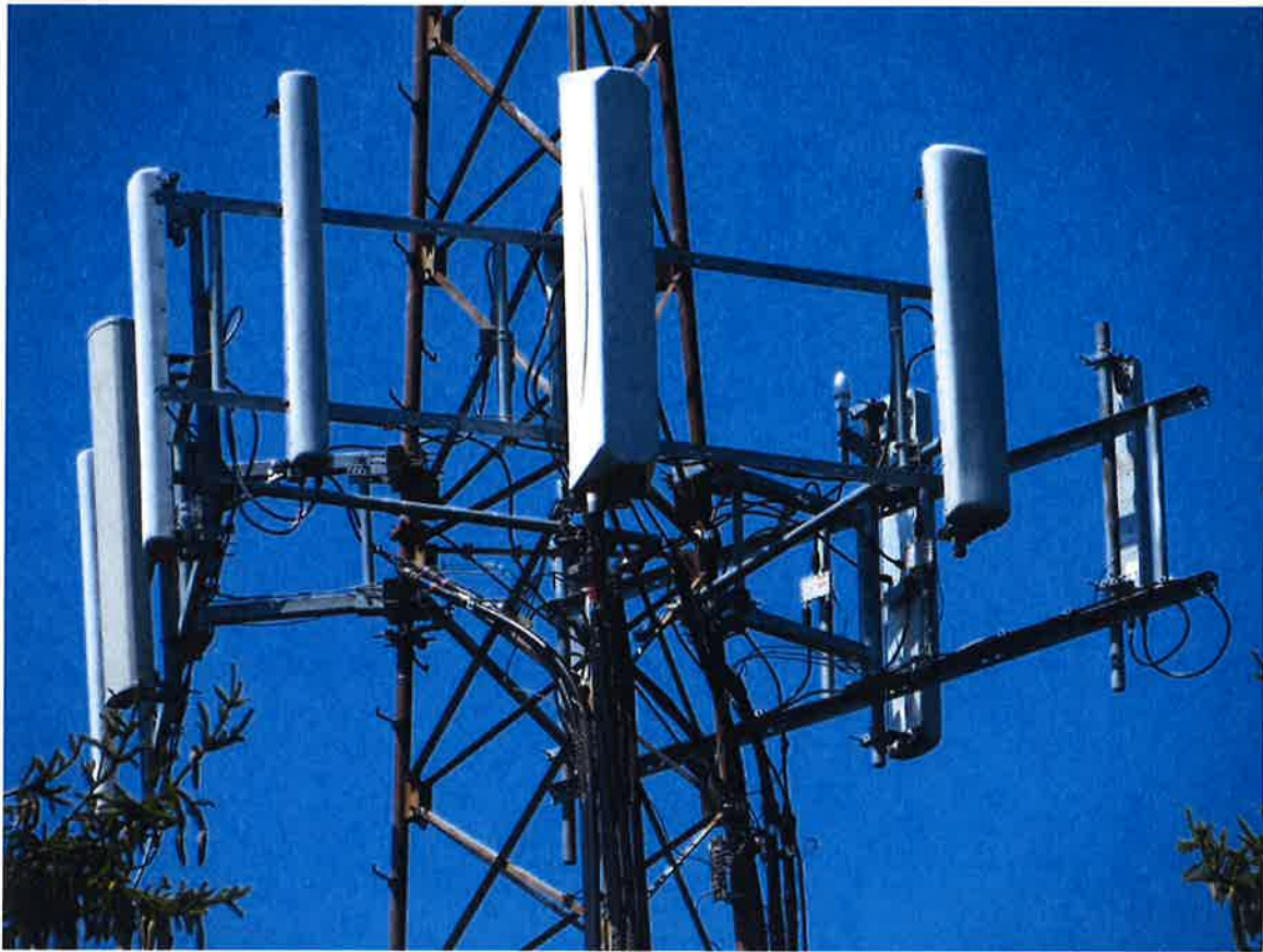
Photo 1: Photo illustrating the Tower with Appurtenances shown.
