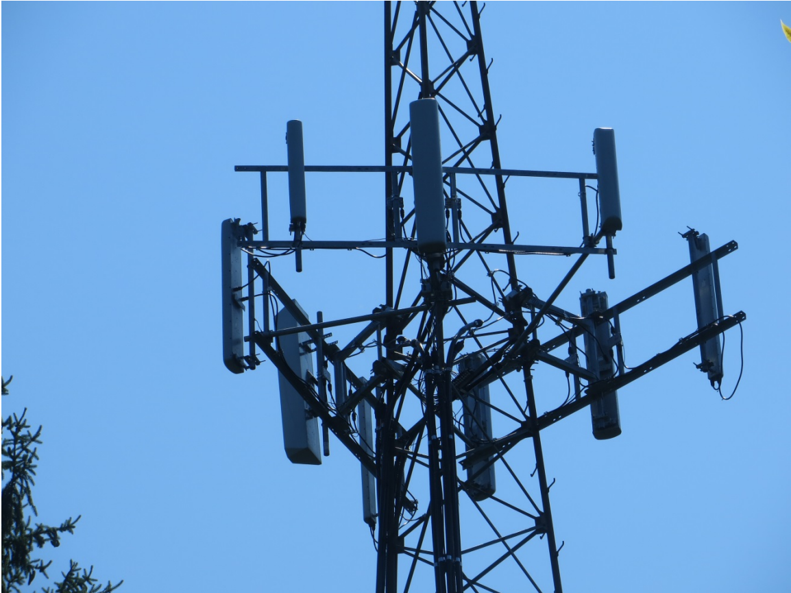
Photo 1: Photo illustrating the Tower with Appurtenances shown.
