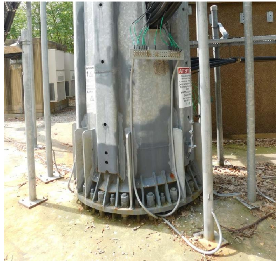
TOWER BASE/FOUNDATION PHOTO
