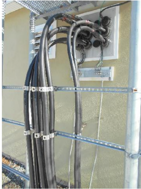
Photos of Verizon's existing cable entry ports and ground bar at shelter.
