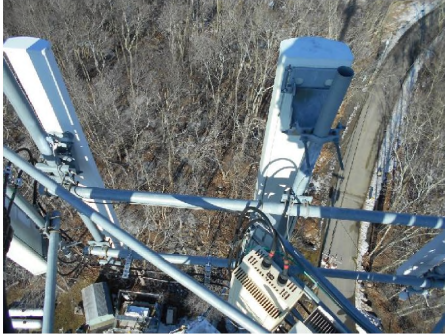
Additional photos of Verizon's typical existing equipment and mounts at 155'.
