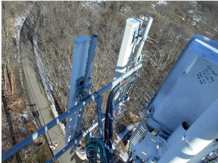
Additional photos of Verizon's typical existing equipment and mounts at 155'.
