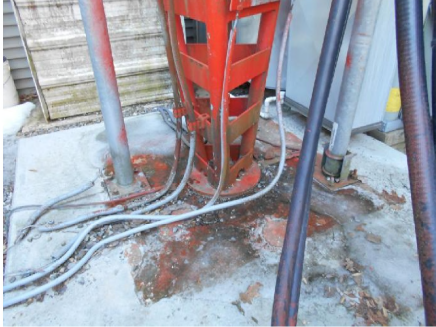
Photo of typical existing base foundation.
