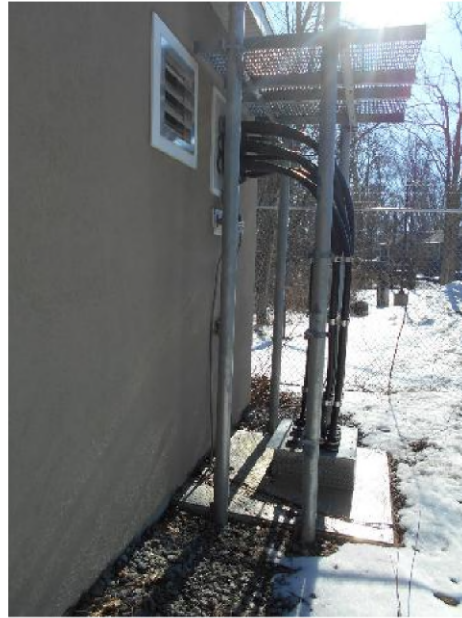
Photo of Verizon's existing ice bridge.
