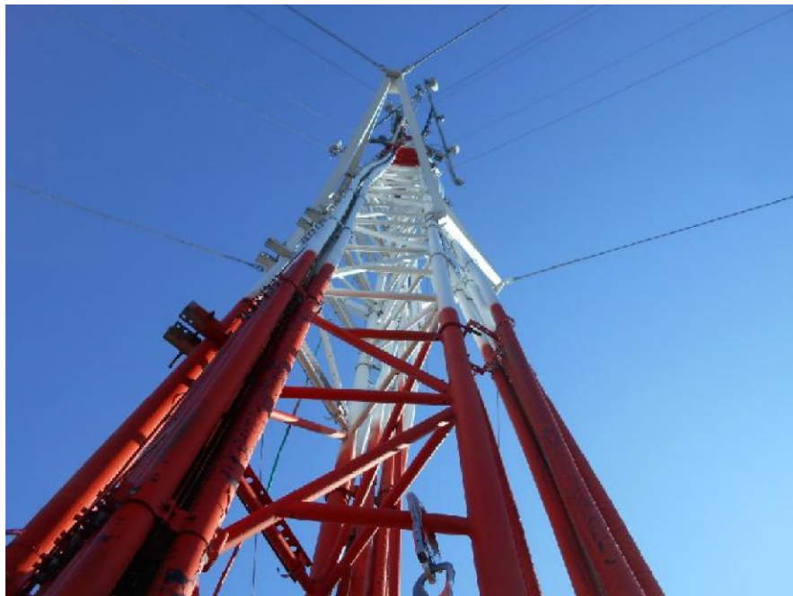
Photos of typical existing guy pull-offs.
