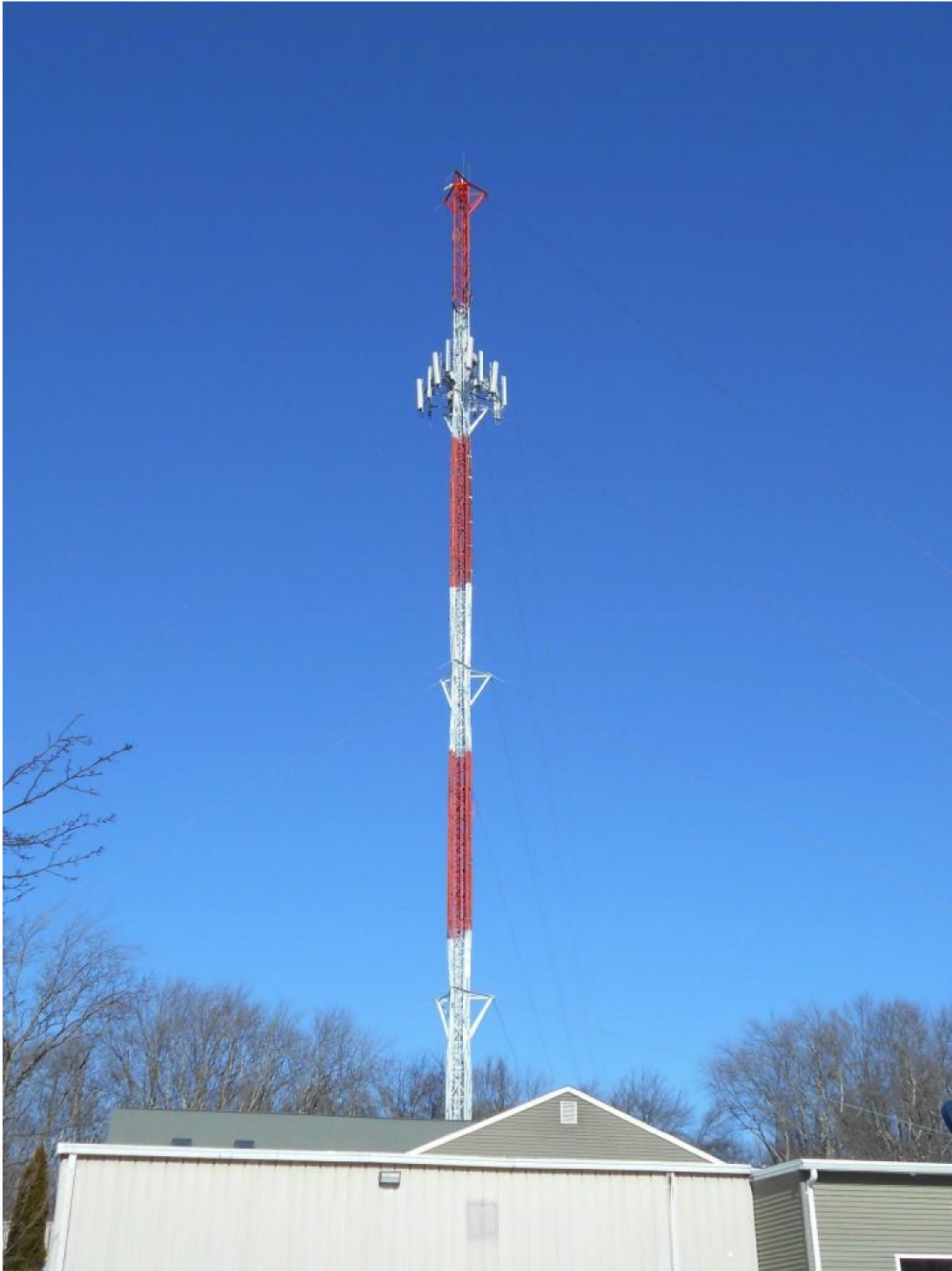
Overview photo of the existing 200' guyed tower located in Prospect, Connecticut.
