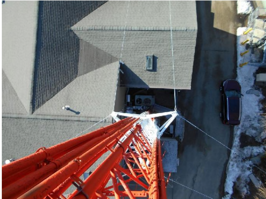
Photos of typical existing guy pull-offs.
