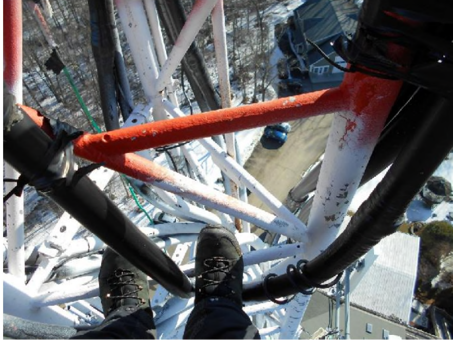
Photos of inactive feed lines taped to tower leg.
