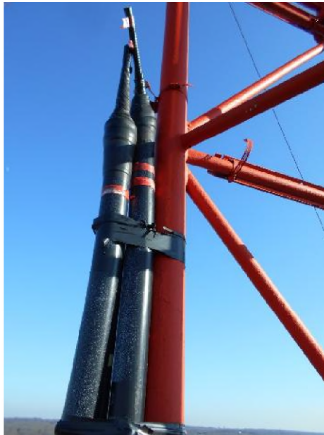
Photos of inactive feed lines taped to tower leg.
