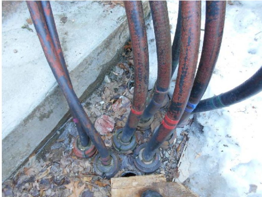
Photo of existing cable entry ports.
