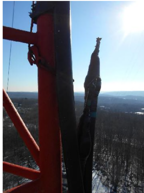
Photos of inactive feed lines taped to tower leg.
