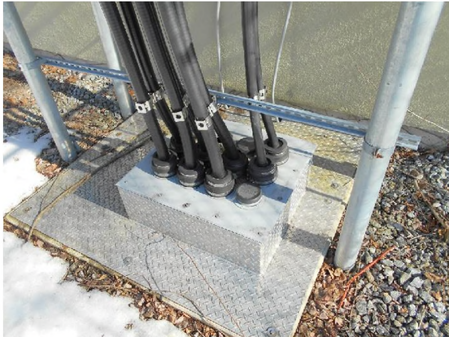
Photos of Verizon's existing cable entry ports and ground bar at shelter.
