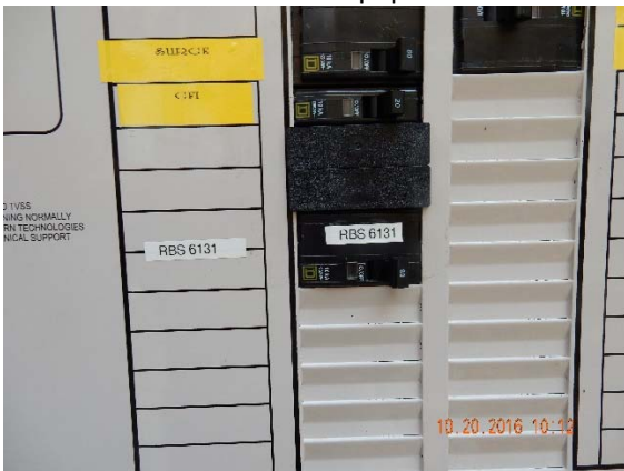
50A Breaker Removed – AFTER (Contractor Photo)
