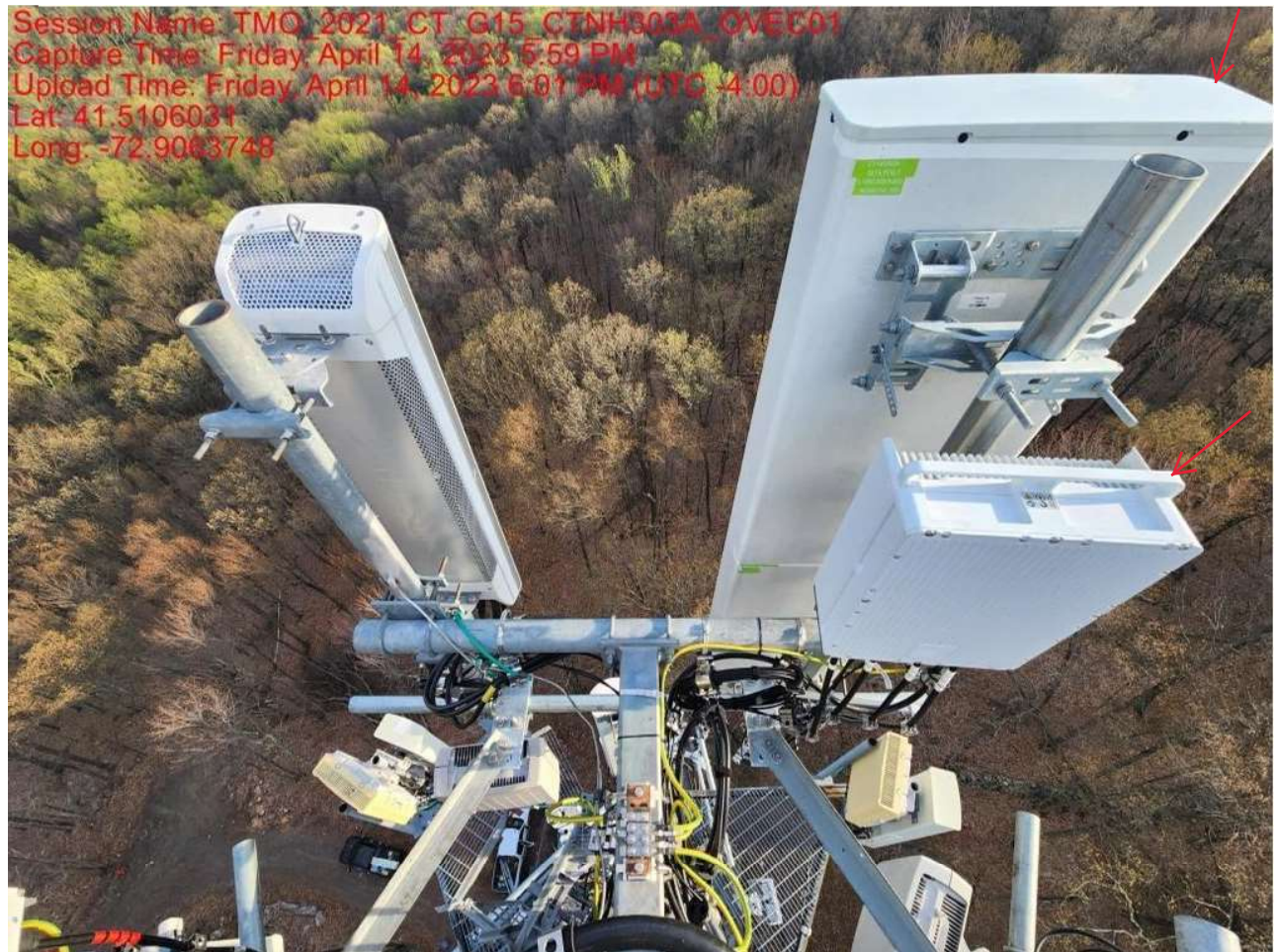
Beta Sector: (1) New Antenna & (1) New RRH Mounted To Existing T-Arm Mount
