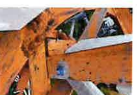
CT-1680 Site Photos (136)
