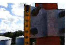
CT-1680 Site Photos (412)
