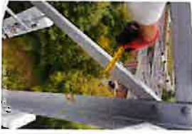
CT-1680 Site Photos (106)
