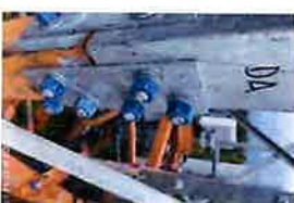
CT-1680 Site Photos (123)
