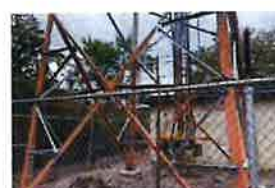
CT-1680 Site Photos (23)
