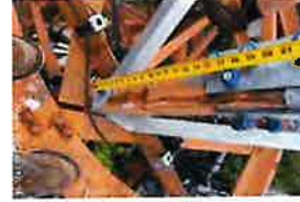
CT-1680 Site Photos (168)
