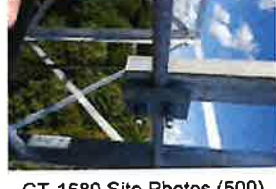
CT-1680 Site Photos (500)
