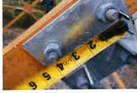
CT-1680 Site Photos (357)
