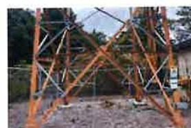
CT-1680 Site Photos (22)
