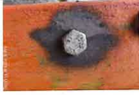
CT-1680 Site Photos (73)
