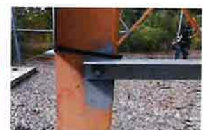
CT-1680 Site Photos (255)
