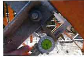
CT-1680 Site Photos (383)
