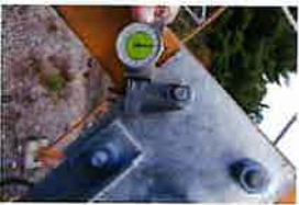
CT-1680 Site Photos (331)
