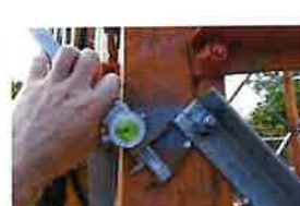
CT-1680 Site Photos (312)
