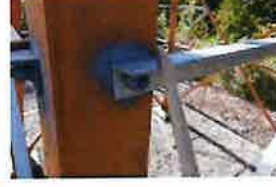
CT-1680 Site Photos (374)
