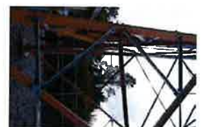
CT-1680 Site Photos (535)
