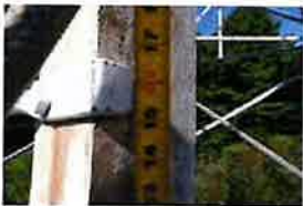
CT-1680 Site Photos (397)
