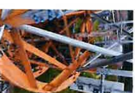
CT-1680 Site Photos (138)
