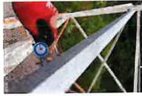
CT-1680 Site Photos (86)
