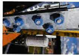
CT-1680 Site Photos (458)
