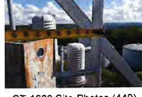
CT-1680 Site Photos (440)
