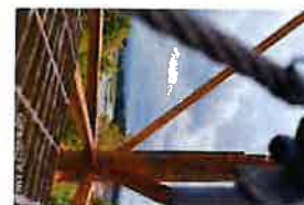
CT-1680 Site Photos (179)
