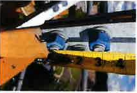
CT-1680 Site Photos (461)
