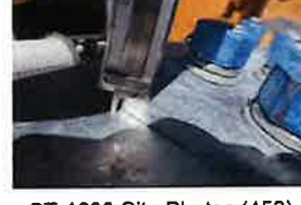
CT-1680 Site Photos (453)
