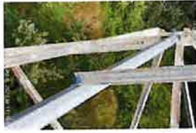
CT-1680 Site Photos (81)
