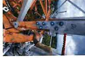
CT-1680 Site Photos (158)
