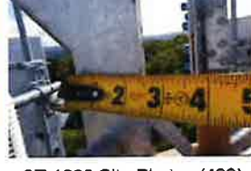
CT-1680 Site Photos (439)
