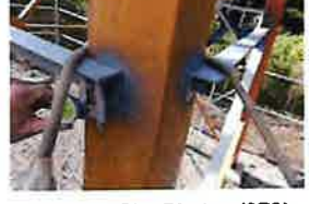
CT-1680 Site Photos (370)
