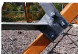
CT-1680 Site Photos (258)
