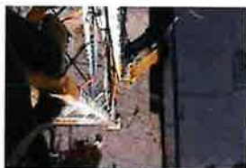
CT-1680 Site Photos (398)
