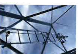
CT-1680 Site Photos (137)
