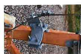
CT-1680 Site Photos (32)
