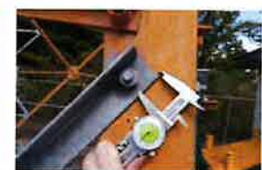
CT-1680 Site Photos (250)
