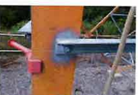
CT-1680 Site Photos (342)
