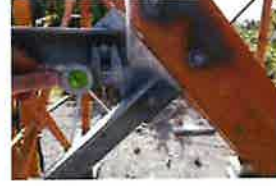
CT-1680 Site Photos (379)
