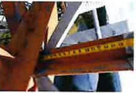
CT-1680 Site Photos (466)
