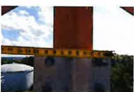
CT-1680 Site Photos (408)
