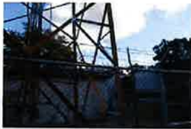
CT-1680 Site Photos (532)
