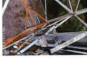
CT-1680 Site Photos (74)
