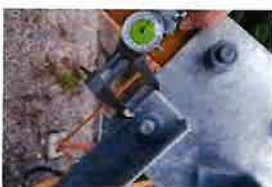
CT-1680 Site Photos (333)
