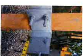
CT-1680 Site Photos (204)
