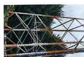
CT-1680 Site Photos (27)
