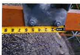
CT-1680 Site Photos (264)
