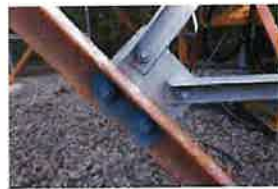
CT-1680 Site Photos (232)
