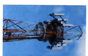
CT-1680 Site Photos (195)
