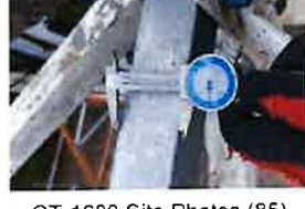
CT-1680 Site Photos (85)
