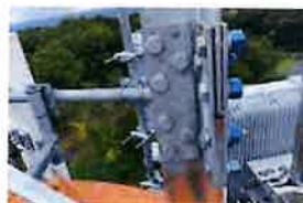
CT-1680 Site Photos (183)
