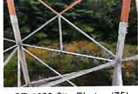
CT-1680 Site Photos (75)
