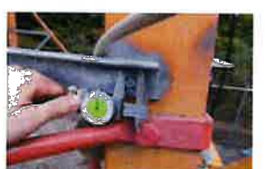
CT-1680 Site Photos (340)
