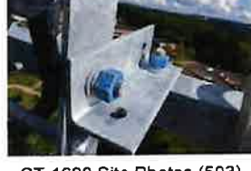
CT-1680 Site Photos (503)
