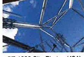
CT-1680 Site Photos (434)
