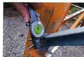
CT-1680 Site Photos (324)
