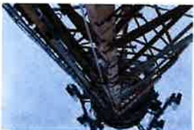
CT-1680 Site Photos (187)
