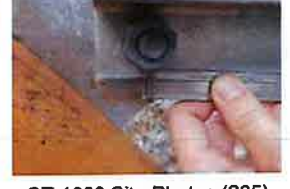
CT-1680 Site Photos (285)
