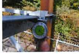
CT-1680 Site Photos (368)
