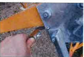
CT-1680 Site Photos (337)
