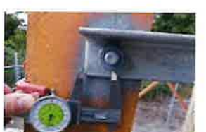
CT-1680 Site Photos (345)
