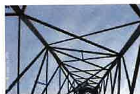
CT-1680 Site Photos (18)
