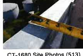
CT-1680 Site Photos (513)
