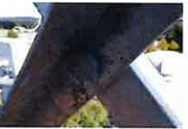
CT-1680 Site Photos (476)
