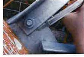
CT-1680 Site Photos (235)
