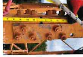
CT-1680 Site Photos (92)
