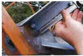
CT-1680 Site Photos (291)
