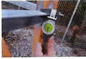
CT-1680 Site Photos (282)
