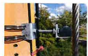
CT-1680 Site Photos (400)
