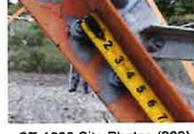
CT-1680 Site Photos (289)
