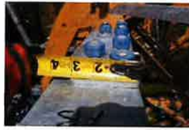
CT-1680 Site Photos (457)
