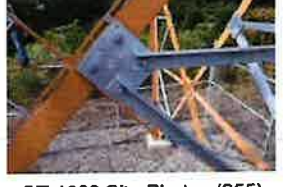
CT-1680 Site Photos (355)
