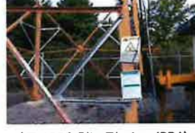
CT-1680 Site Photos (224)
