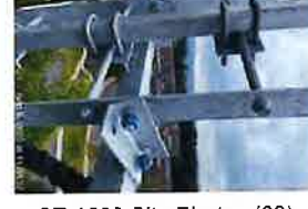
CT-1680 Site Photos (99)
