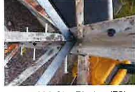
CT-1680 Site Photos (79)
