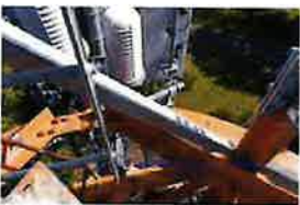
CT-1680 Site Photos (472)
