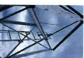
CT-1680 Site Photos (133)
