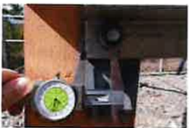
CT-1680 Site Photos (257)
