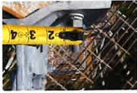
CT-1680 Site Photos (426)
