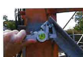
CT-1680 Site Photos (311)
