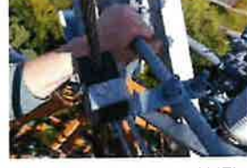
CT-1680 Site Photos (447)
