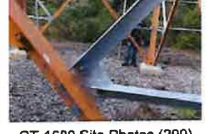
CT-1680 Site Photos (290)
