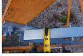
CT-1680 Site Photos (358)
