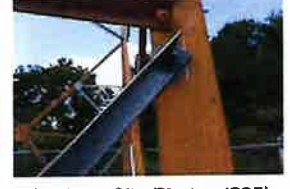
CT-1680 Site Photos (295)
