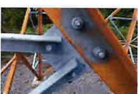
CT-1680 Site Photos (349)
