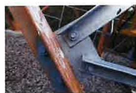
CT-1680 Site Photos (243)
