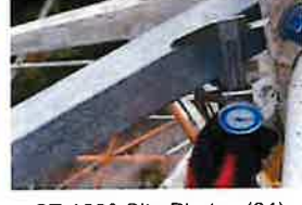
CT-1680 Site Photos (84)
