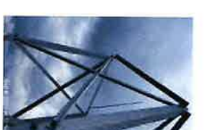
CT-1680 Site Photos (140)
