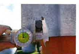
CT-1680 Site Photos (416)
