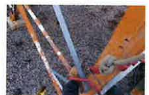
CT-1680 Site Photos (325)
