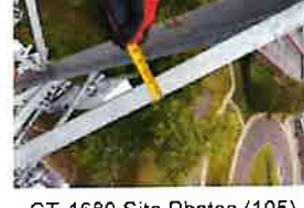
CT-1680 Site Photos (105)
