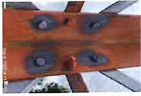
CT-1680 Site Photos (72)
