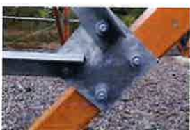
CT-1680 Site Photos (263)
