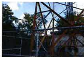
CT-1680 Site Photos (533)
