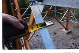
CT-1680 Site Photos (359)
