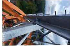
CT-1680 Site Photos (162)
