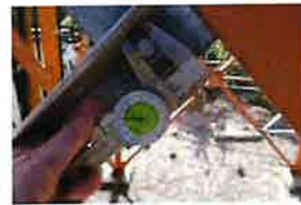
CT-1680 Site Photos (382)
