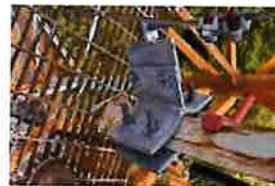
CT-1680 Site Photos (178)
