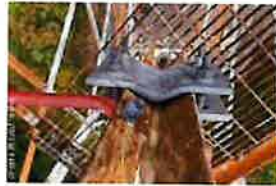
CT-1680 Site Photos (177)
