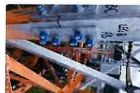
CT-1680 Site Photos (184)
