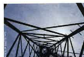
CT-1680 Site Photos (19)
