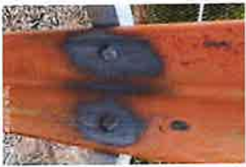
CT-1680 Site Photos (71)
