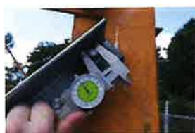
CT-1680 Site Photos (296)
