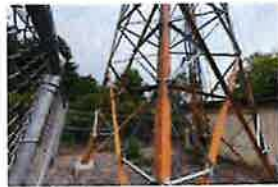
CT-1680 Site Photos (11)
