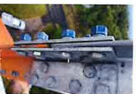
CT-1680 Site Photos (126)
