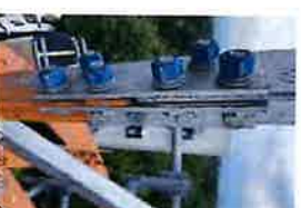
CT-1680 Site Photos (132)
