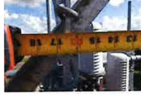
CT-1680 Site Photos (441)
