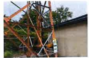
CT-1680 Site Photos (10)
