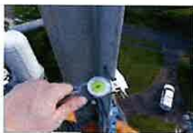
CT-1680 Site Photos (468)
