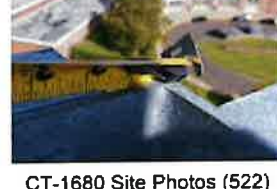
CT-1680 Site Photos (522)
