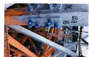
CT-1680 Site Photos (185)
