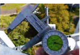
CT-1680 Site Photos (488)
