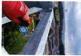
CT-1680 Site Photos (107)
