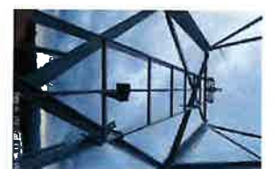
CT-1680 Site Photos (115)
