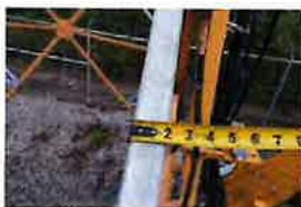
CT-1680 Site Photos (328)
