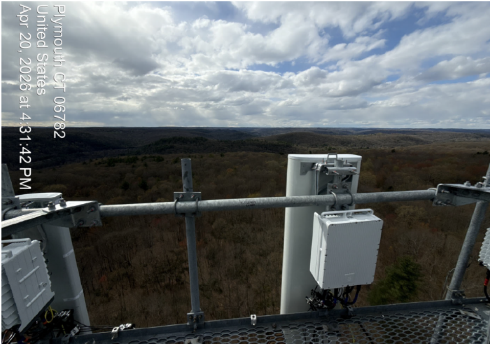
Gamma sector antennas and RRHs installed on existing mount
