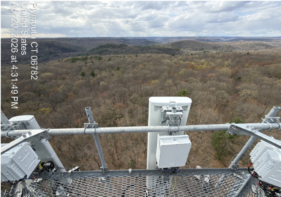
Gamma sector antennas and RRHs installed on existing mount
