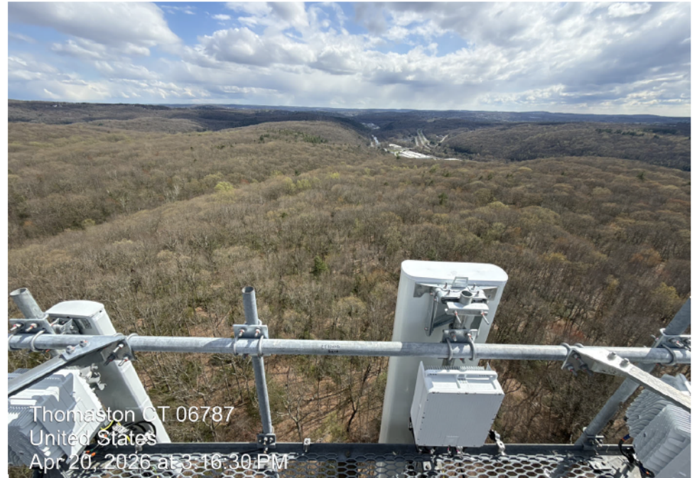
Beta sector antennas and RRHs installed on existing mount
