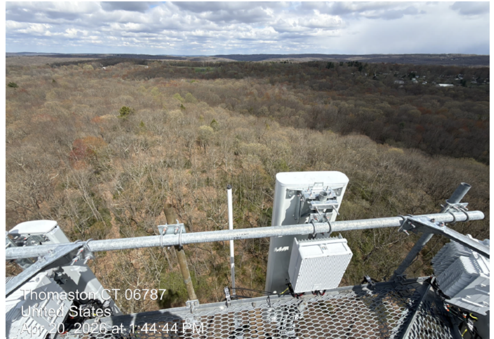
Alpha sector antennas and RRHs installed on existing mount
