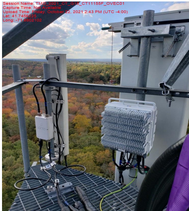
Sector 3 Mount Reinforced Assembly (10/22/2021)
