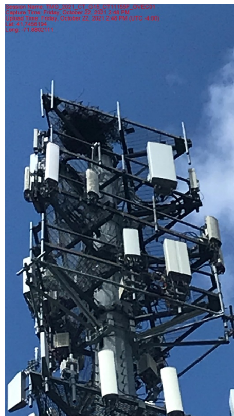
2 nd Mount from the top Reinforced Assembly (10/22/2021)
