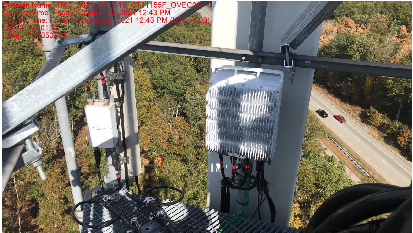
Sector 1 Mount Reinforced Assembly (10/22/2021)
