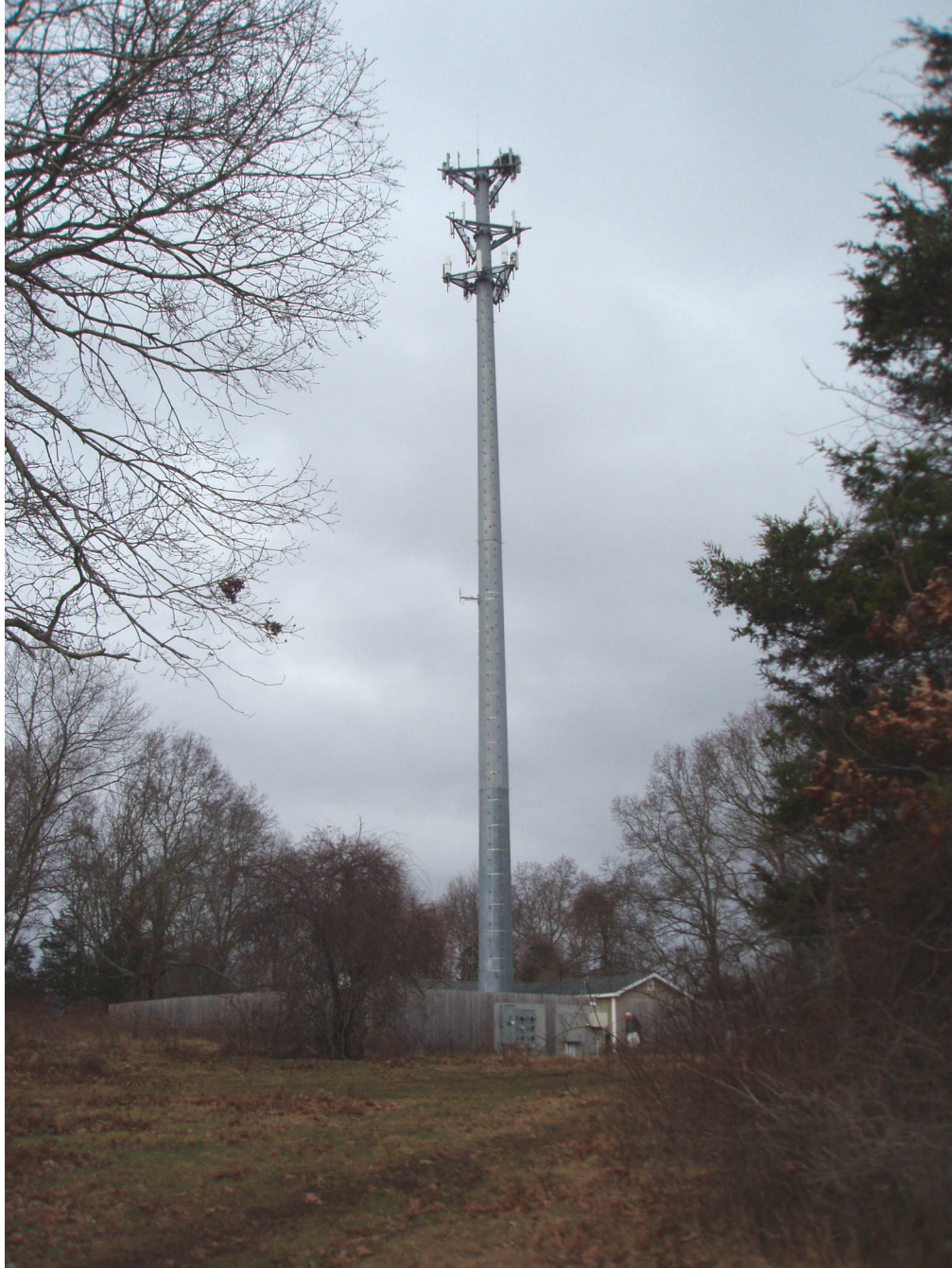
View of existing tower
