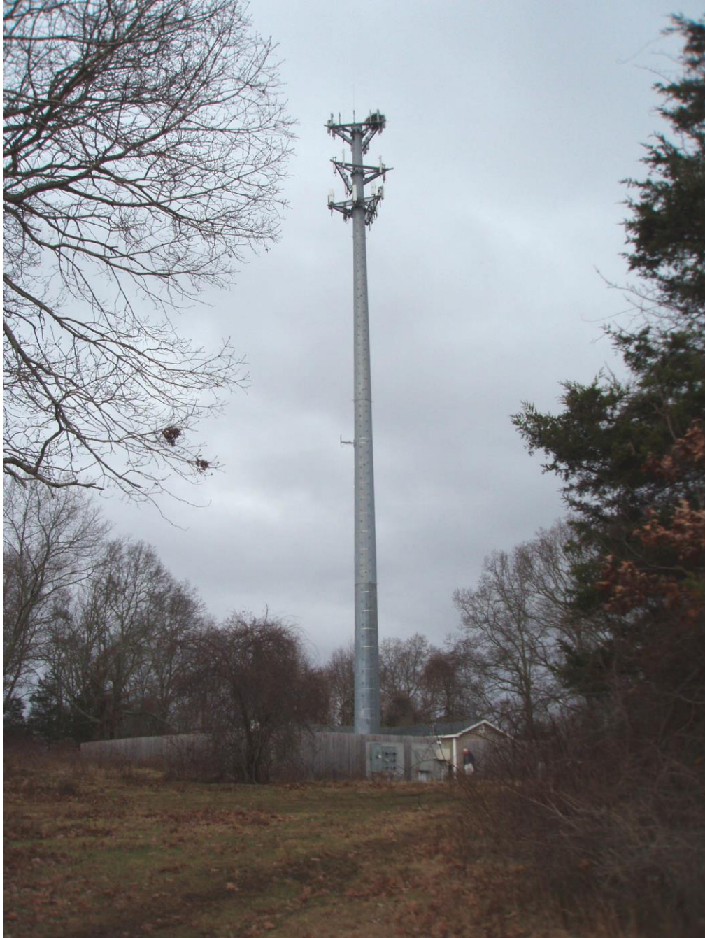
View of existing tower
