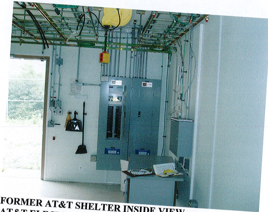
FORMER AT&T SHELTER FOR BASE STATION & ASSOCIATED EQUIPMENT DECOMMISSIONED
