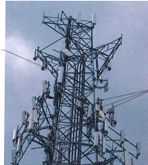
EXIST (2) 1900MHz RRH AND (1) 800MHz RRH STACK MOUNTED ON EXIST MOUNT TO BE RELOCATED (TYP PER SECTOR)
