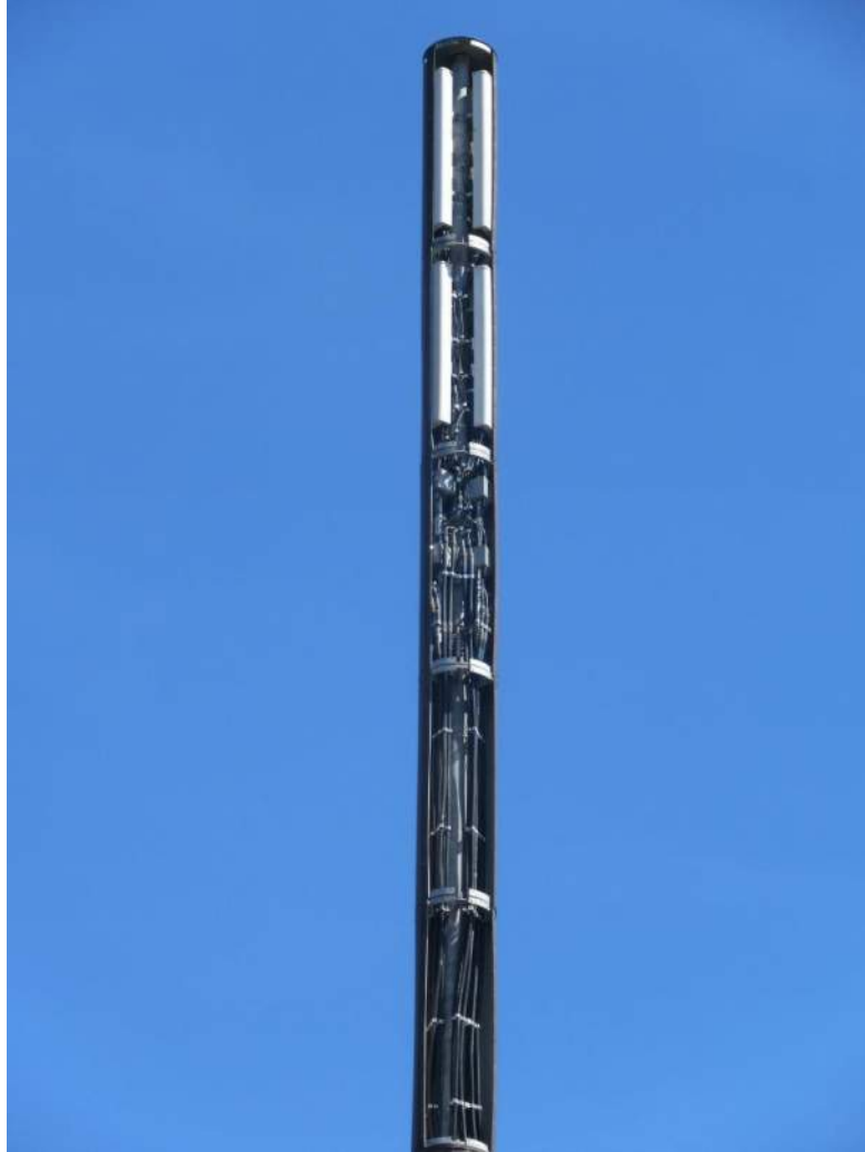
Photo 1: Photo illustrating the tower with appurtenances shown.
