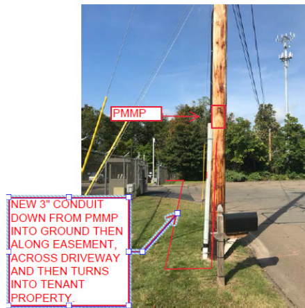
CONDUIT PATH FROM PMMP TO NEW FIBER J-BOX
