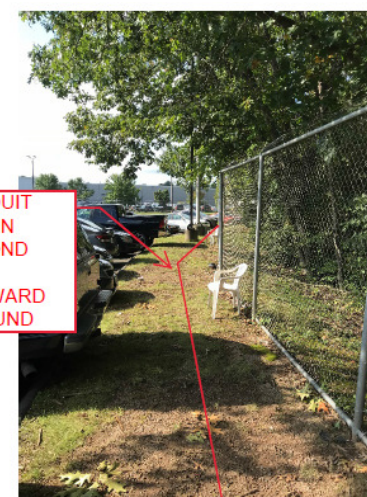
CONDUIT PATH FROM PMMP TO NEW FIBER J-BOX
