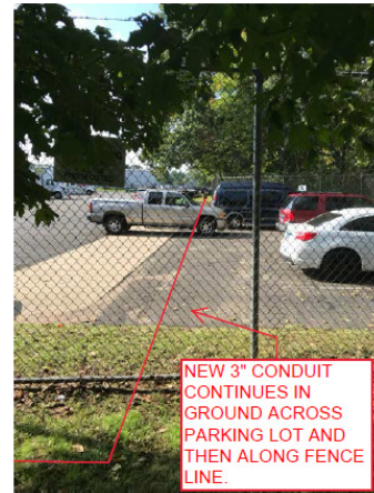
CONDUIT PATH FROM PMMP TO NEW FIBER J-BOX
