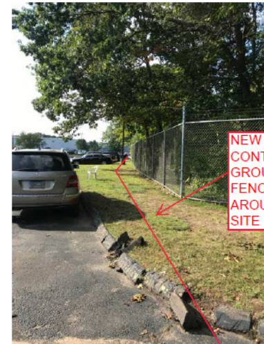
CONDUIT PATH FROM PMMP TO NEW FIBER J-BOX
