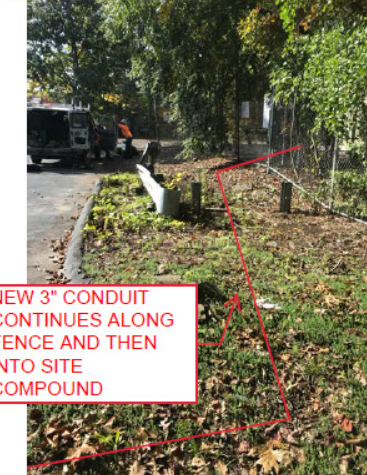
CONDUIT PATH FROM PMMP TO NEW FIBER J-BOX
