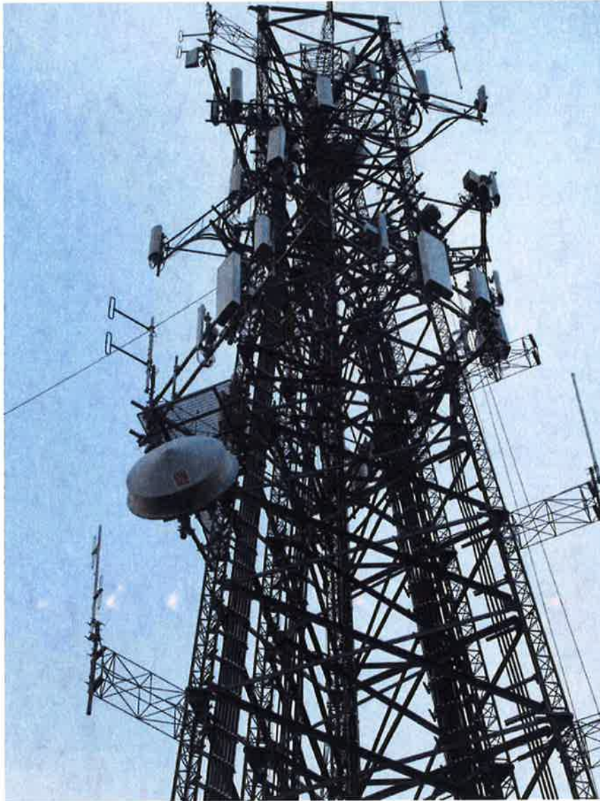
Photo 1: Photo illustrating the Tower with Appurtenances shown.
