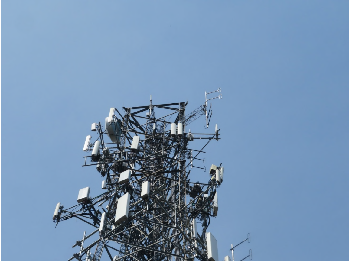
Photo 1: Photo illustrating the Tower with Appurtenances shown.
