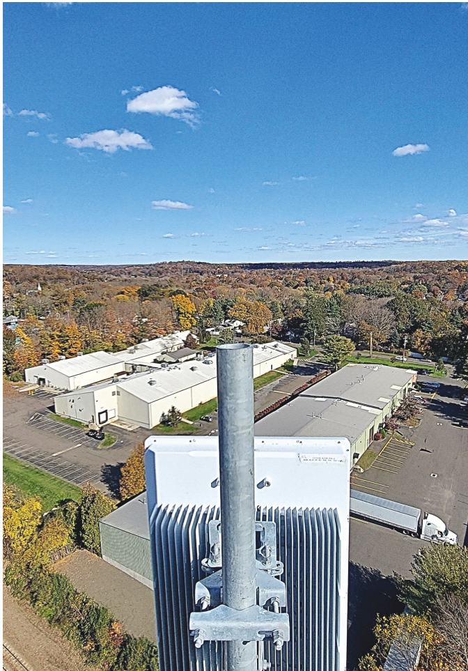
New antenna installed to existing pipe
