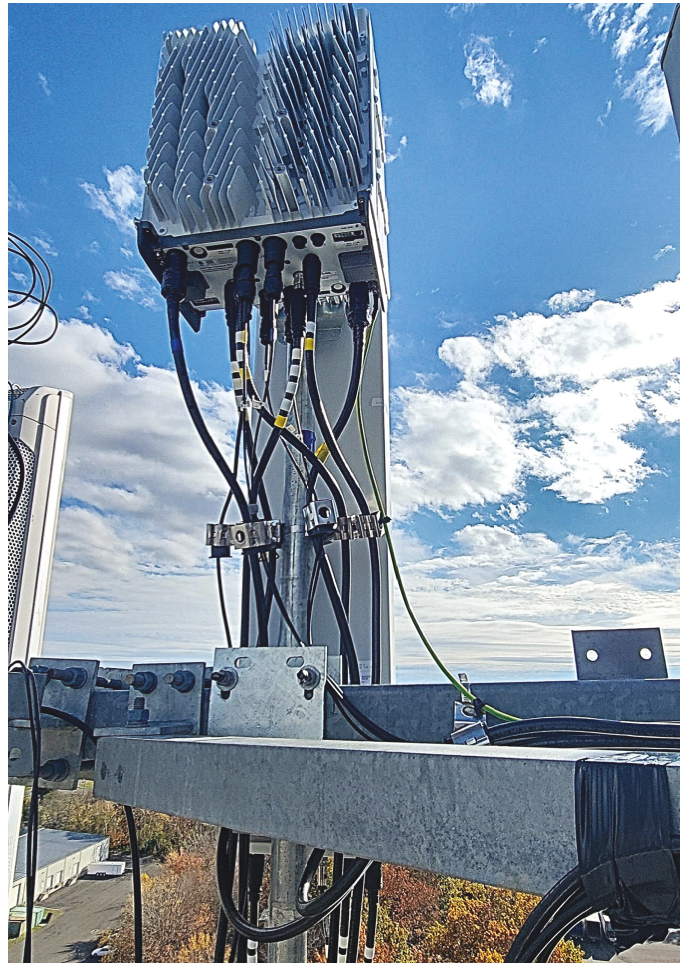
New antenna and RRH installed to existing pipe
