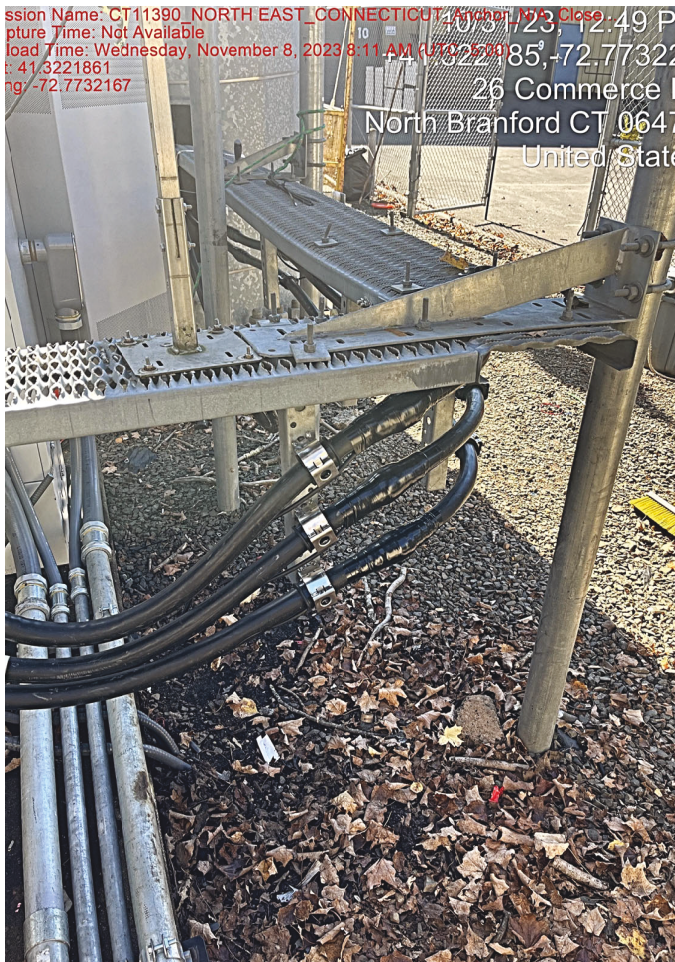
New signal cables installed in existing ice bridge
