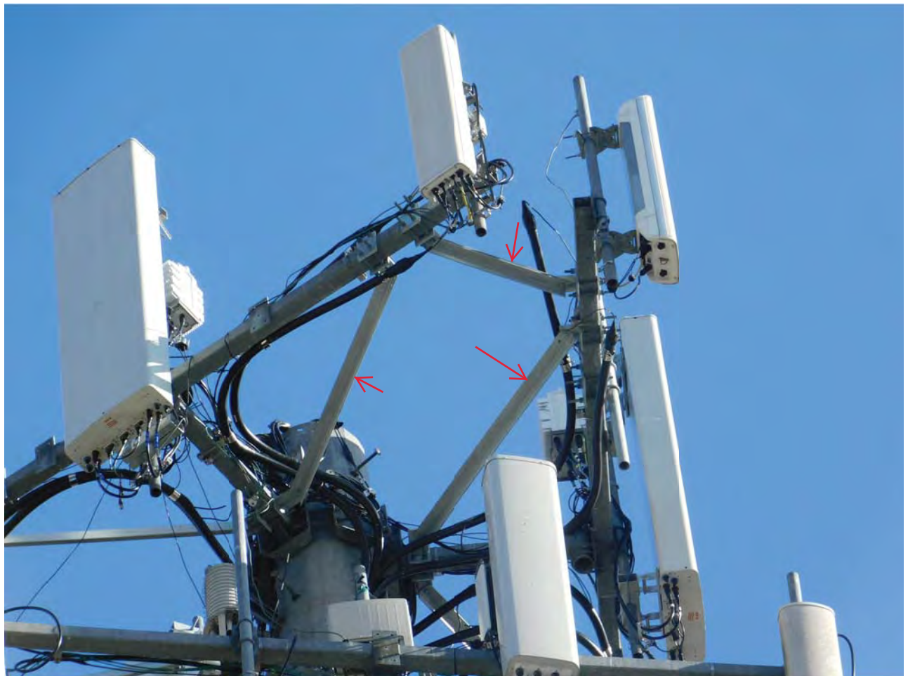
Additional V-Bracing & End Connectors Installed On Existing Sector Frames (Throughout)
