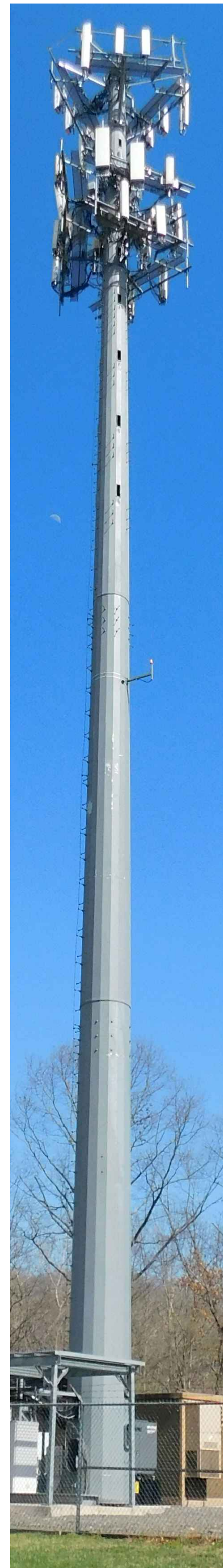
EXISTING TOWER PHOTO N.T.S.
