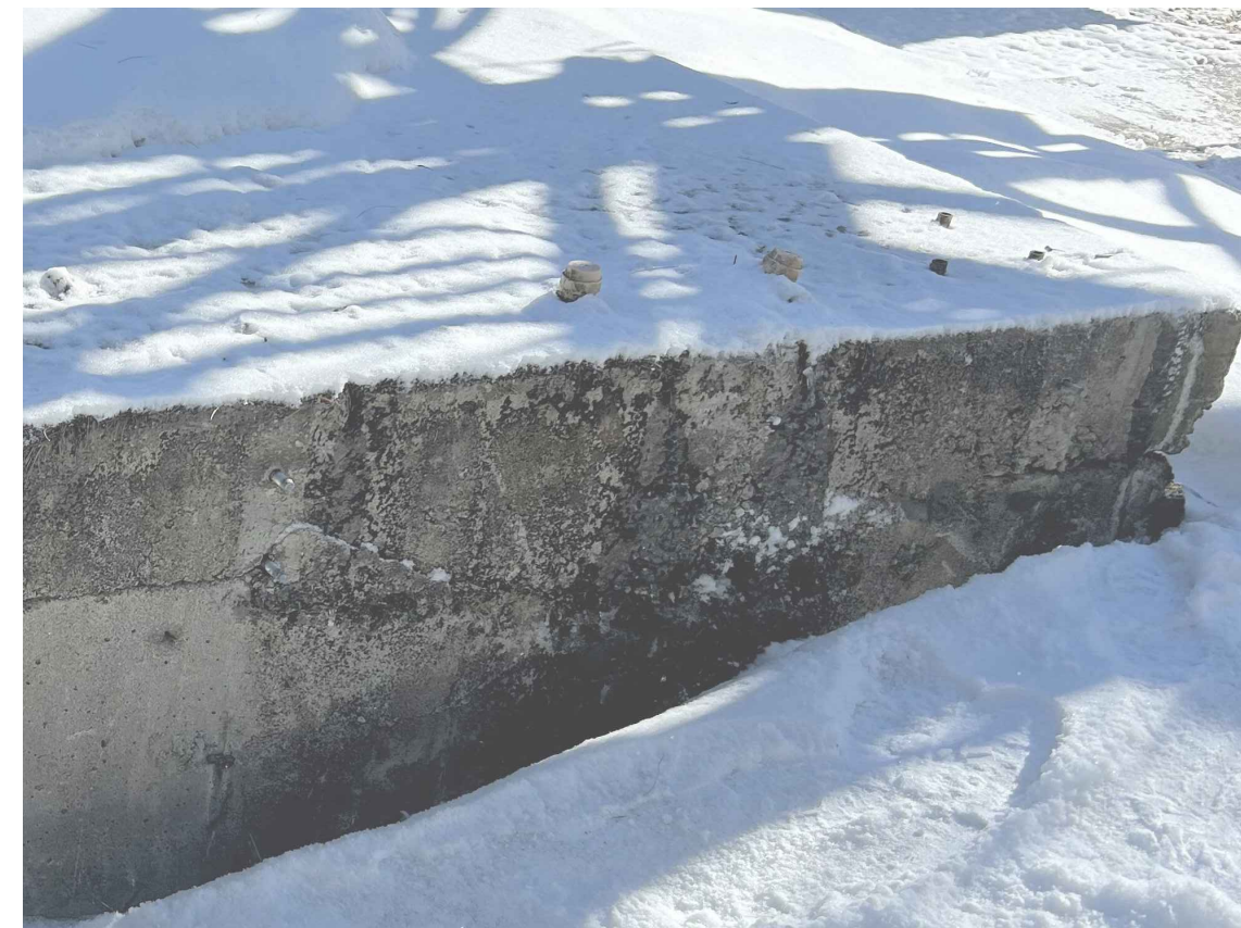
2 MINOR SPALLING
