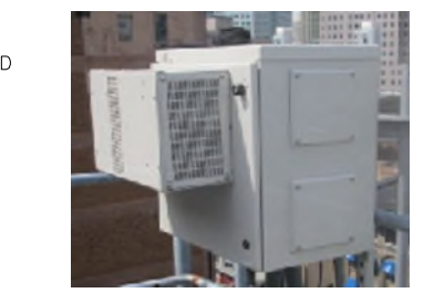
EMERSON NETXTEND COMPACT 2416 CABINET ENCLOSURE: ALUMINUM DIMENSIONS (HxWxD): 24" X 24" X 25.25" WEIGHT: 64LBS (EXCLUDES EQUIPMENT) WEATHER TIGHTNESS: NEMA TYPE 3R
