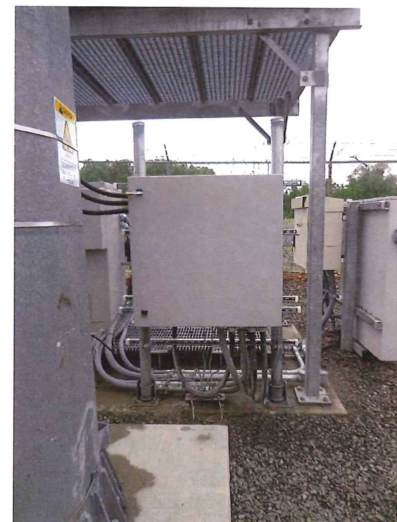
4 A-3 EXIST FIBER DISTRIBUTION BOX SCALE: NTS
