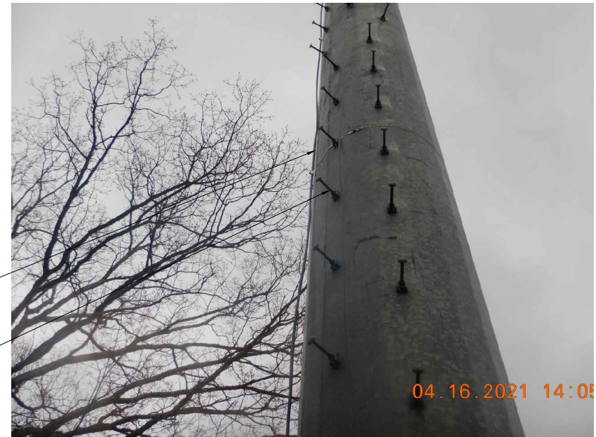
Existing Safety Climb Existing Climbing Facility
