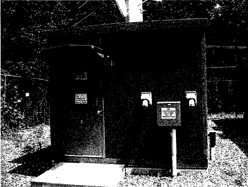
FORMER AT&T SHELTER FOR BASE STATION & ASSOCIATED EQUIPMENT DECOMMISSIONED
