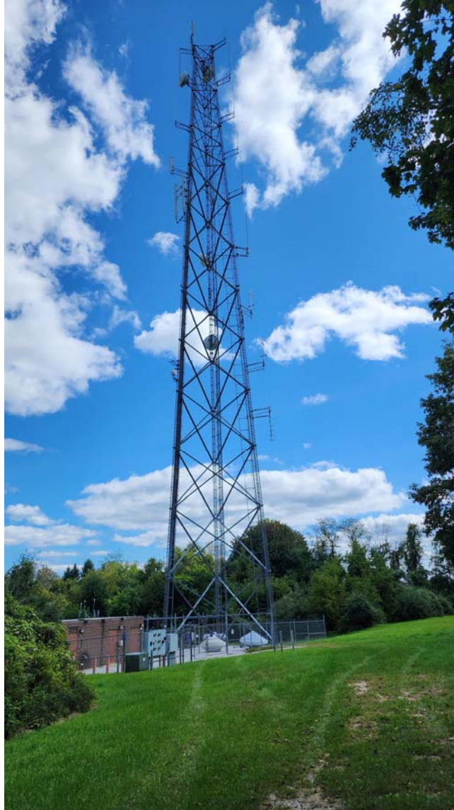
Figure 1: View of ES-074 New Milford
