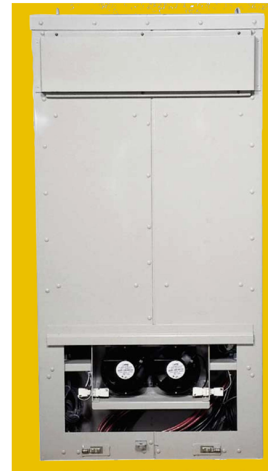
REAR VIEW 60ECv2 BATTERY CABINET (REAR PANEL REMOVED)
