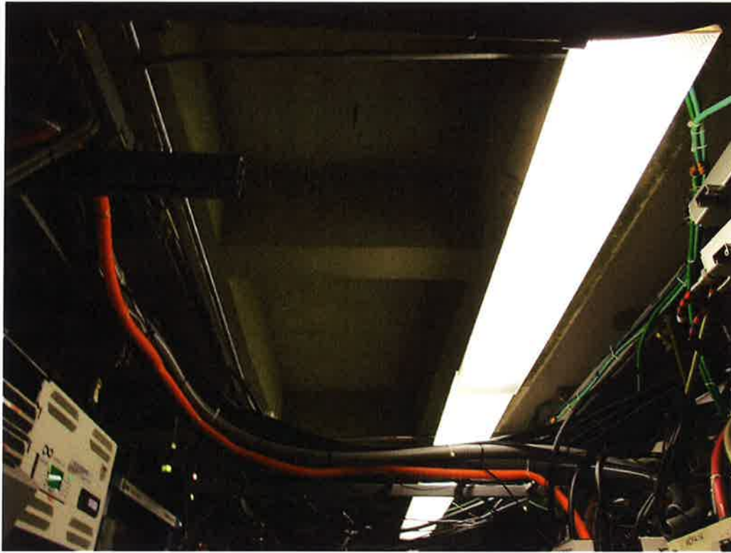
Photo 3: Sample photo illustrating the existing roof construction.
