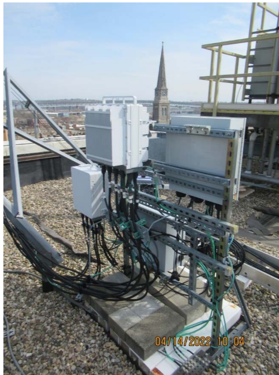
Photo 4: Sample photo illustrating the existing RRH's.
