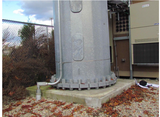
Existing monopole base
