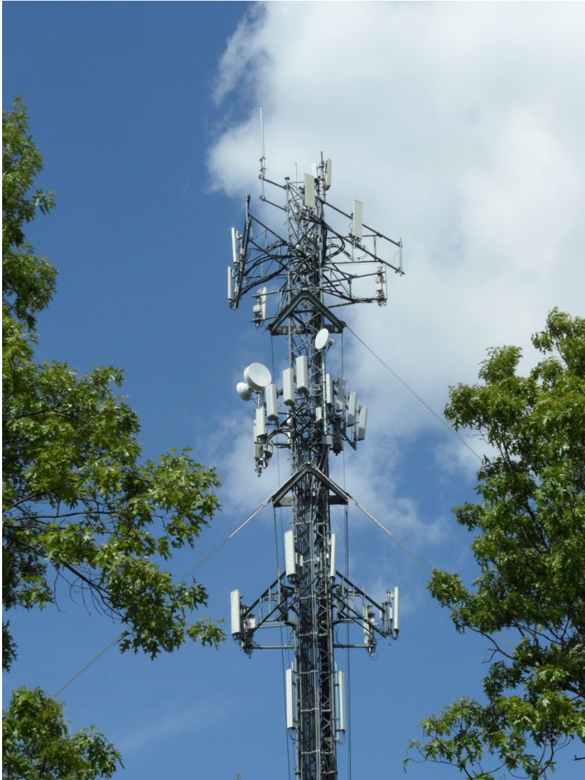
Photo 1: Photo illustrating the Tower with Appurtenances shown.
