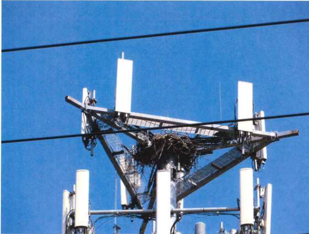
Photo 1: Photo illustrating the Monopole with Appurtenances shown.
