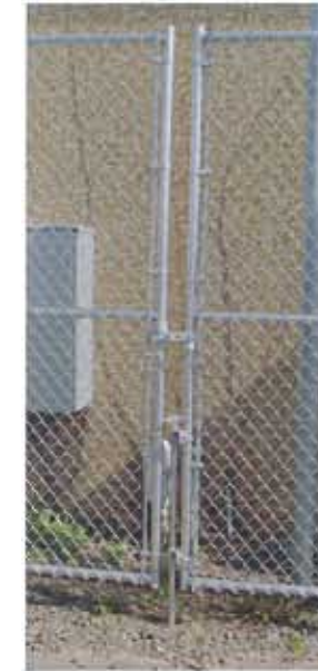
ISSUE #3: NO LOCK ON (2) COMPOUND GATES. RECOMMENDATION: INSTALL LOCKS ON BOTH GATES.
