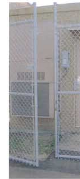
ISSUE #3: NO LOCK ON (2) COMPOUND GATES. RECOMMENDATION: INSTALL LOCKS ON BOTH GATES.
