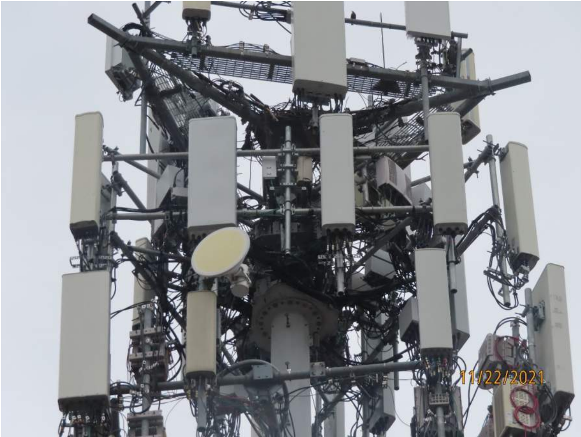
Photo 1: Photo illustrating the Tower with Appurtenances shown.
