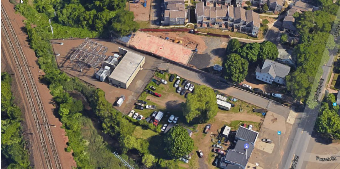
Quinnipiac Substation. 1100 Quinnipiac Ave, New Haven CT 06513 Source: Google Maps 2017
