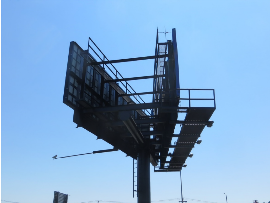
Photo 1: Photo illustrating the monopole with appurtenances shown.
