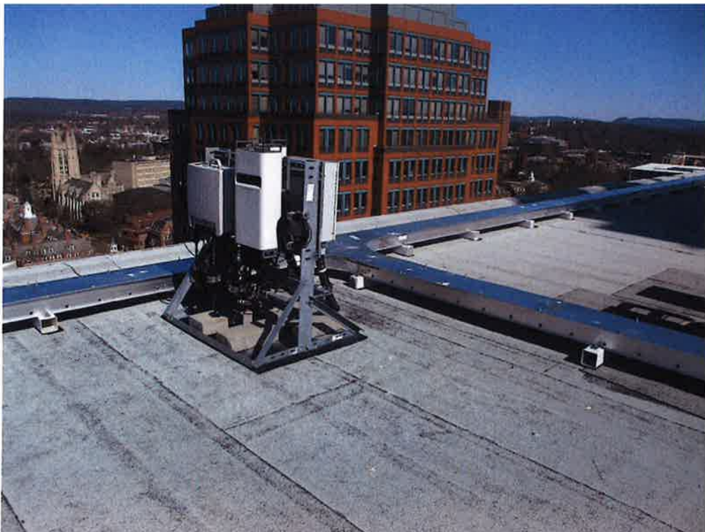
Photo 4: Sample photo illustrating the existing RRH non-penetrating ballast mount.
