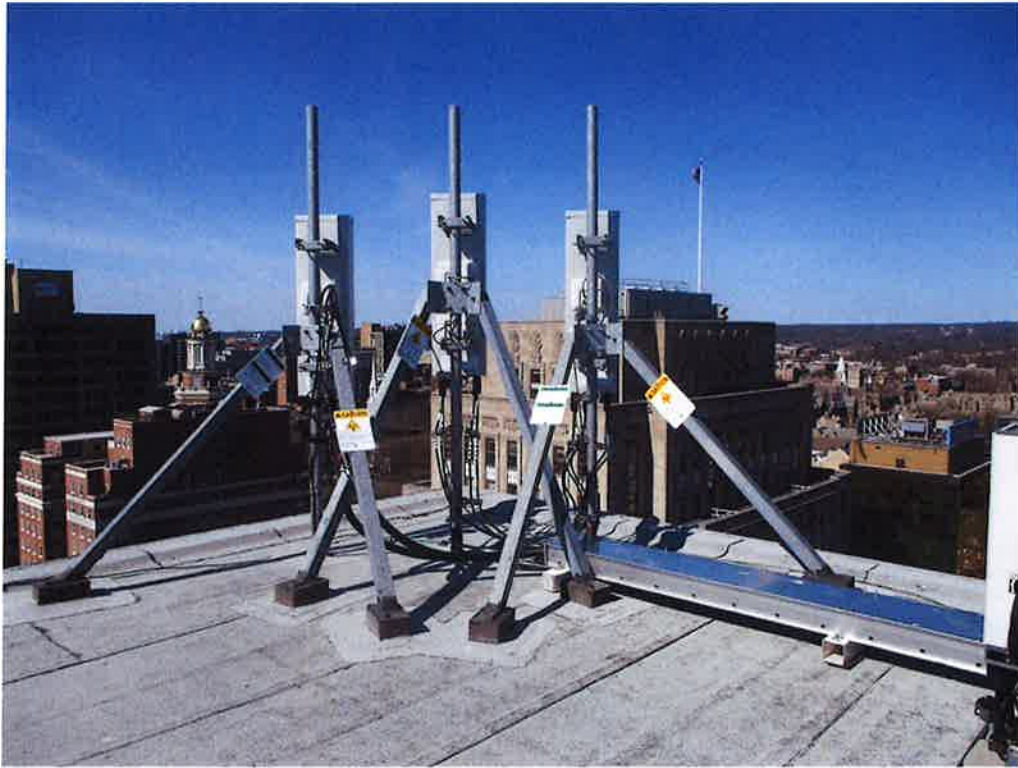
Photo 3: Sample photo illustrating the existing gamma sector mount.
