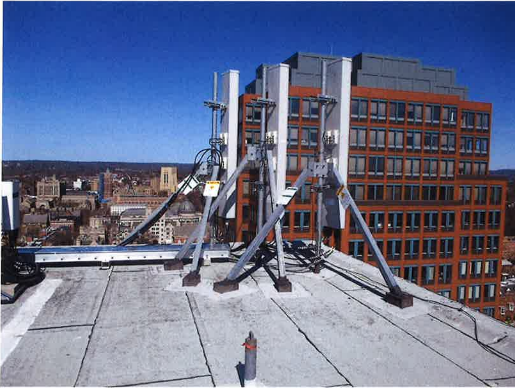
Photo 1: Sample photo illustrating the existing alpha sector mount.
