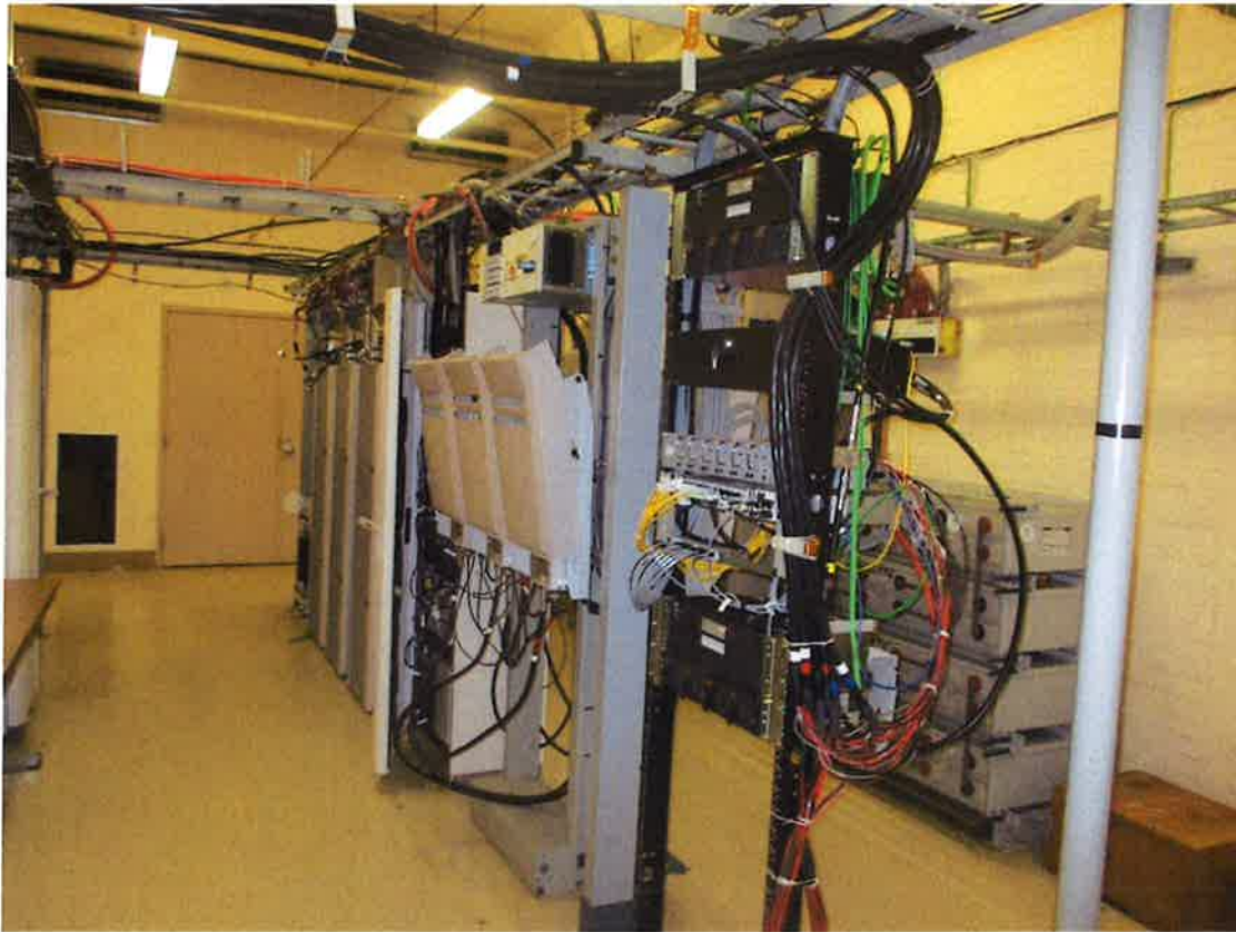
Photo 5: Sample photo illustrating the existing equipment room.
