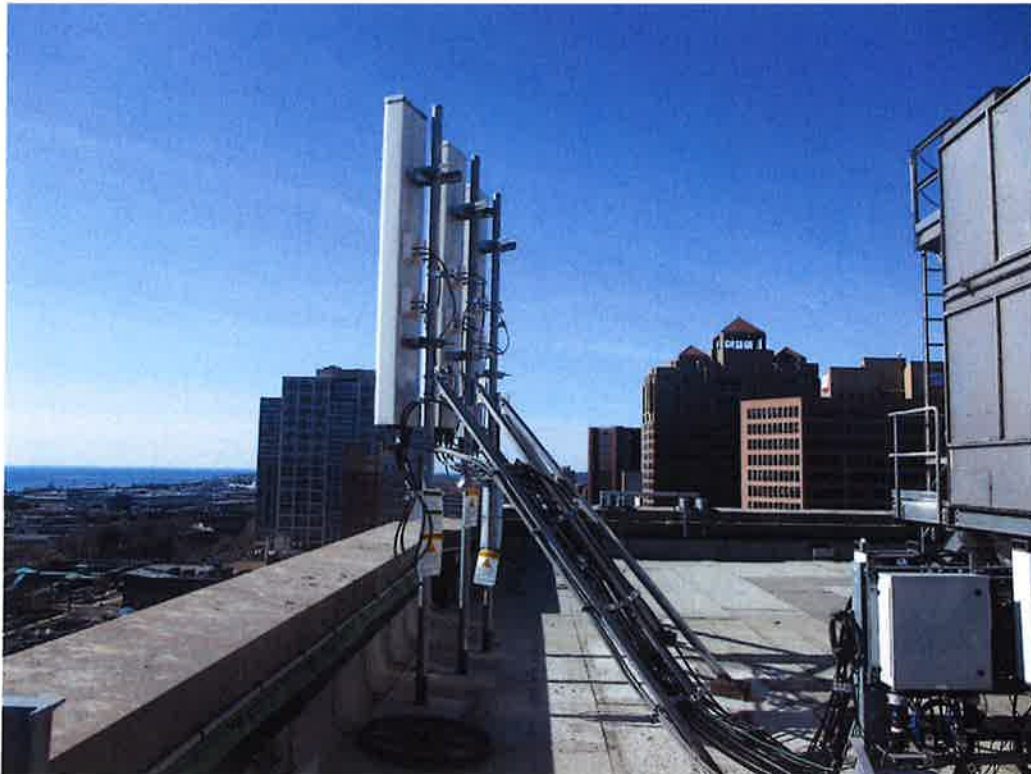
Photo 2: Sample photo illustrating the existing beta sector mount.
