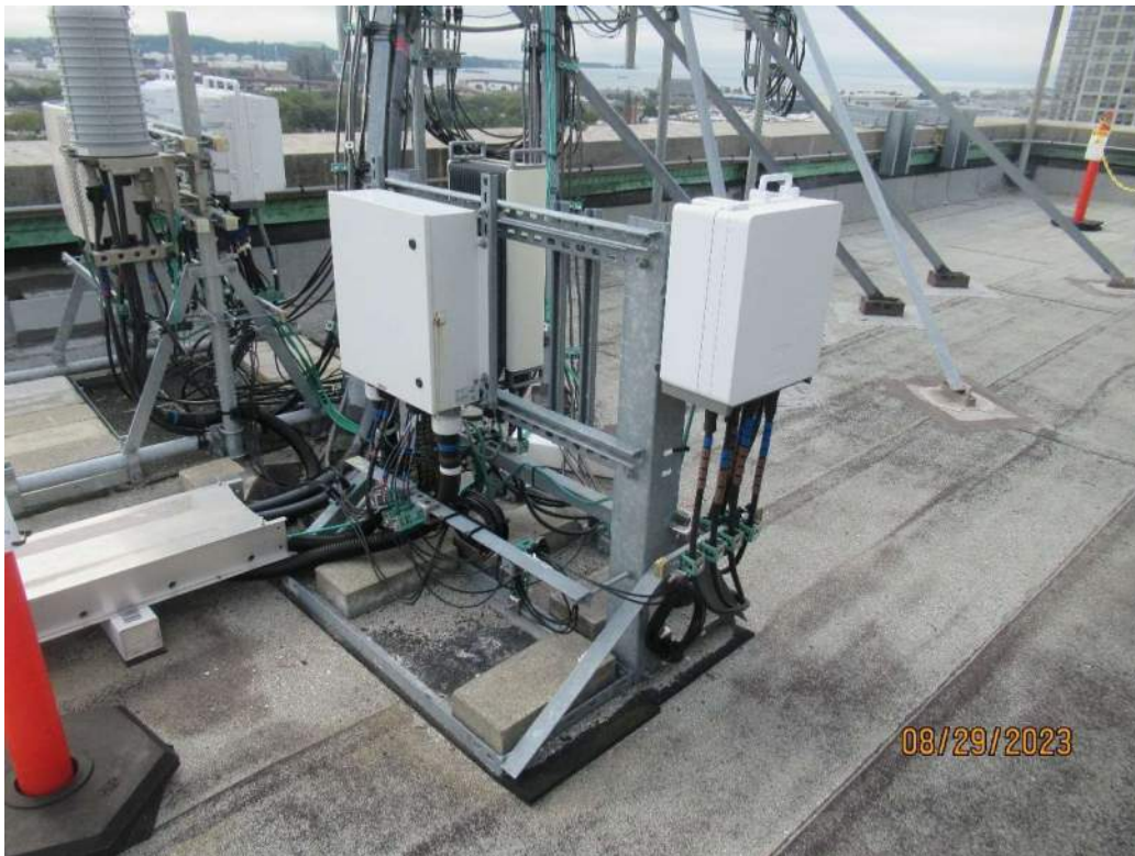
Photo 4: Sample photo illustrating an existing RRH ballast sled at Beta sector.
