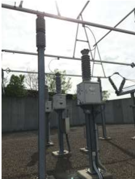
Photos showing the existing CCVT units and one of the junction boxes. Units are at the end of their lifespan. Pictures by UI 2017.
