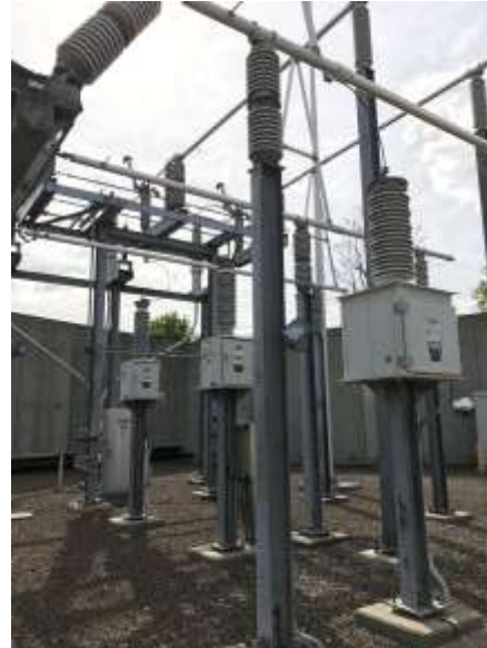
Photos showing the existing CCVT units and one of the junction boxes. Units are at the end of their lifespan. Pictures by UI 2017.
