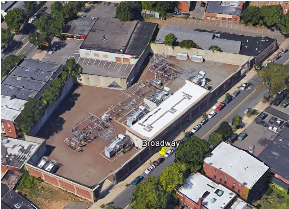
Broadway Substation (56 Goffe Street, New Haven, CT) Google Earth 2016
