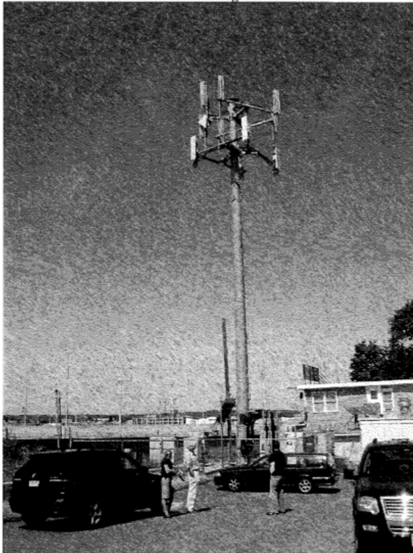
View of Existing Tower
