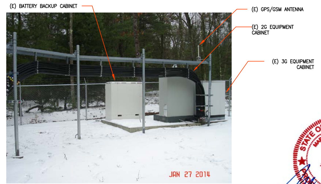
EXISTING EQUIPMENT AREA. N.T.S.
