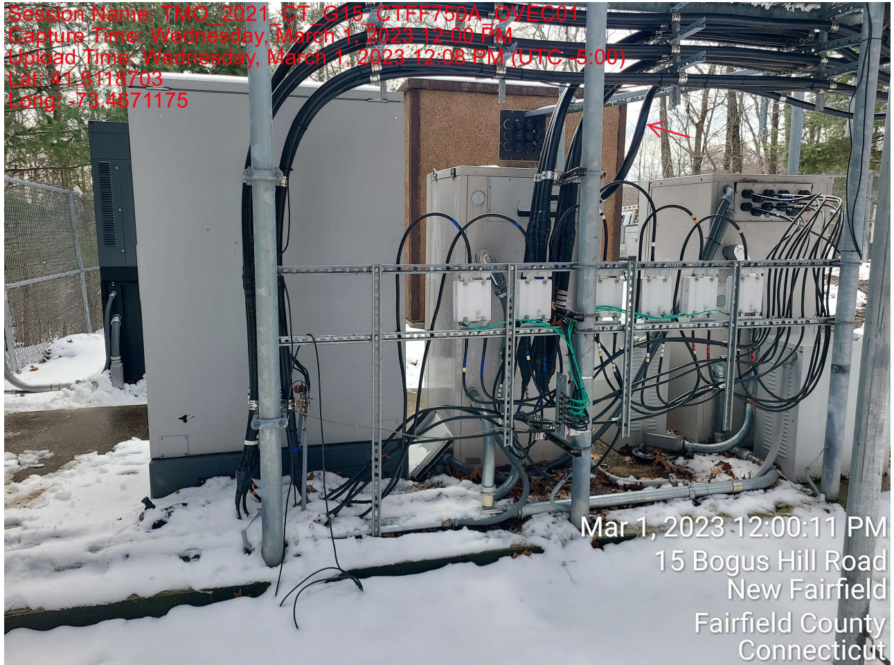
(1) New Signal Cable Run Along The Existing Cable Bridge
