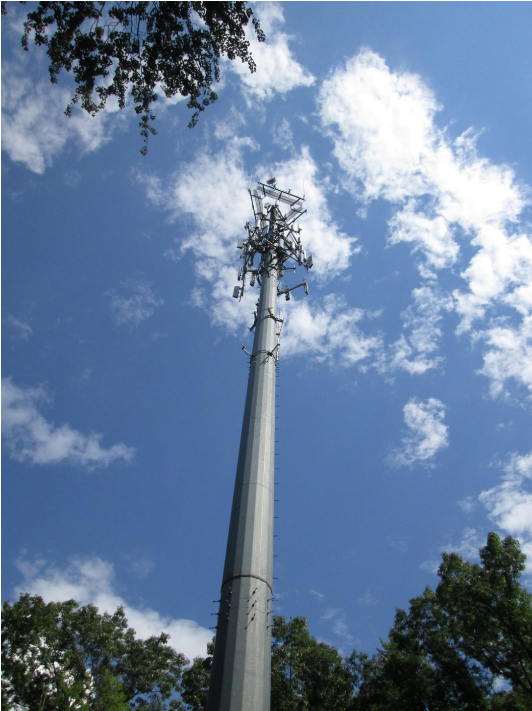
Overview photo of 175' monopole tower.
