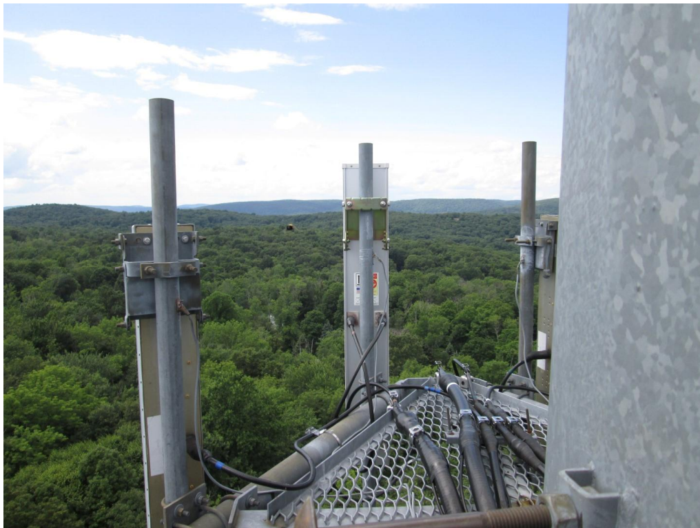
Photos of existing Sprint antennas on platform at 155'.
