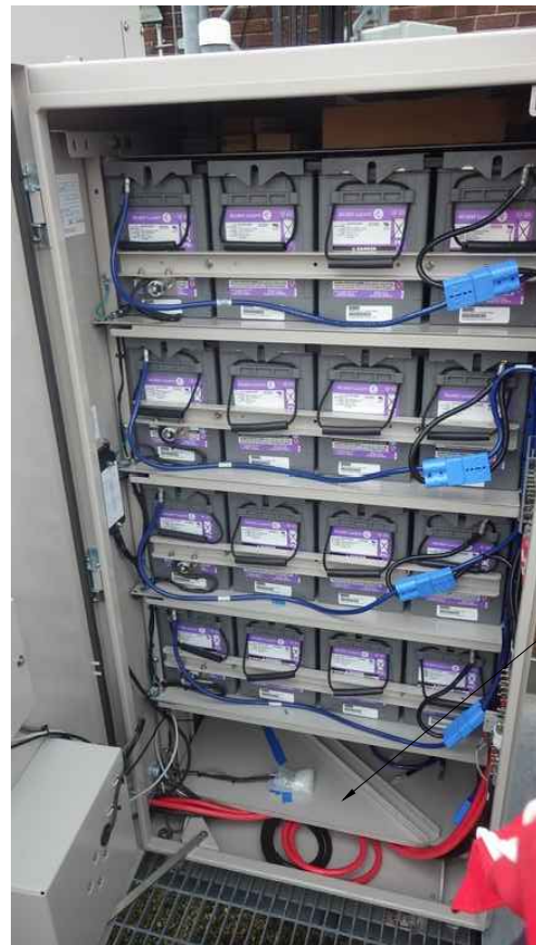
EXISTING BBU CABINET ③ SCALE: NTS
