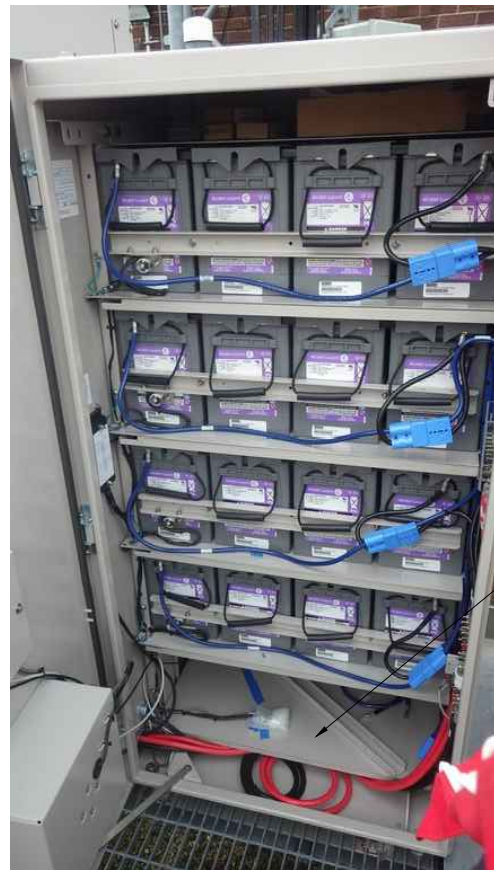
EXISTING BBU CABINET ③ SCALE: NTS
