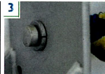
3 Pulling back, rock the tool side-to-side to engage the collapsible washer.
