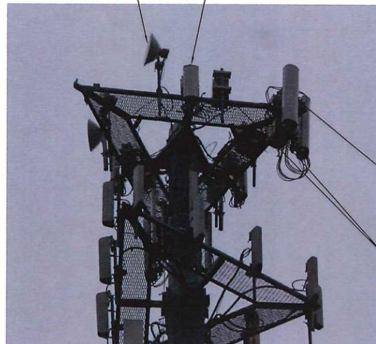
EXIST SPRINT PANEL ANTENNA TO BE RELOCATED TO REPLACEMENT ANTENNA MOUNT (TYP OF 1 PER SECTOR, TOTAL OF 3)
